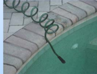
An example of an indirect cross-connection.
