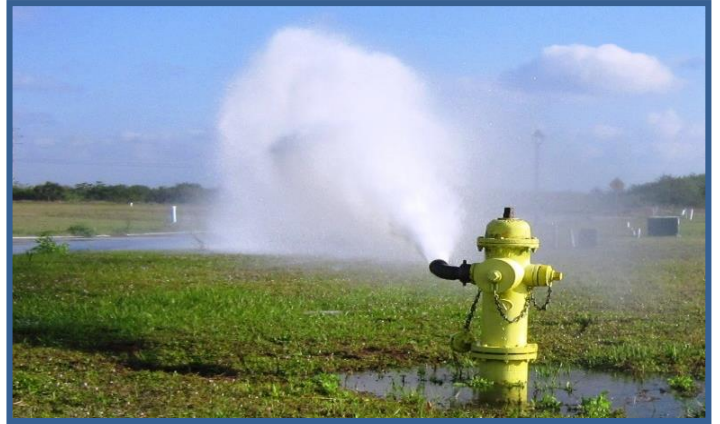
Top image: Unmanned hydrant flushing Left image: Automatic flushing device
