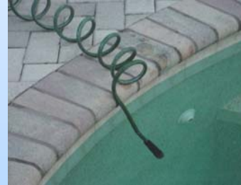
An example of an indirect cross-connection.
